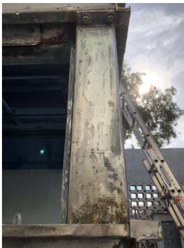
Pictures prep work being done on tower and coating being applied to supports
