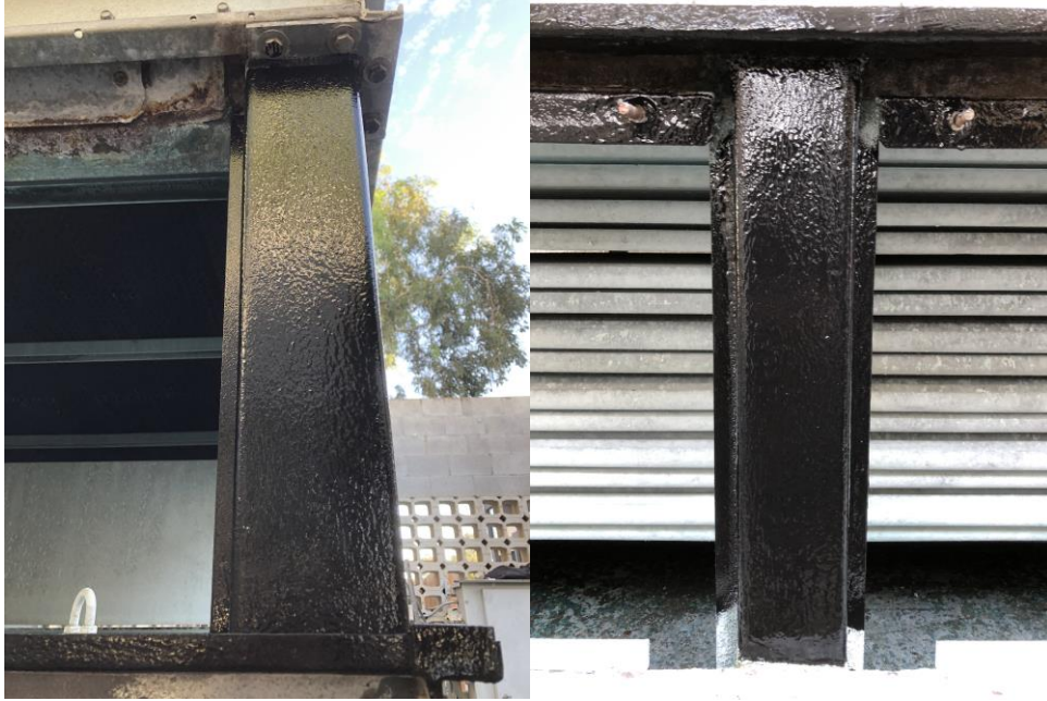
Coating on the supports
