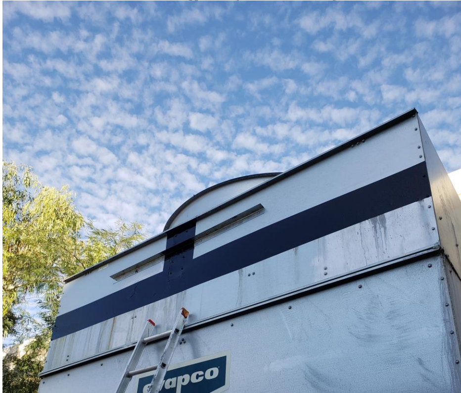
Reinforced upper casing with exterior coating
