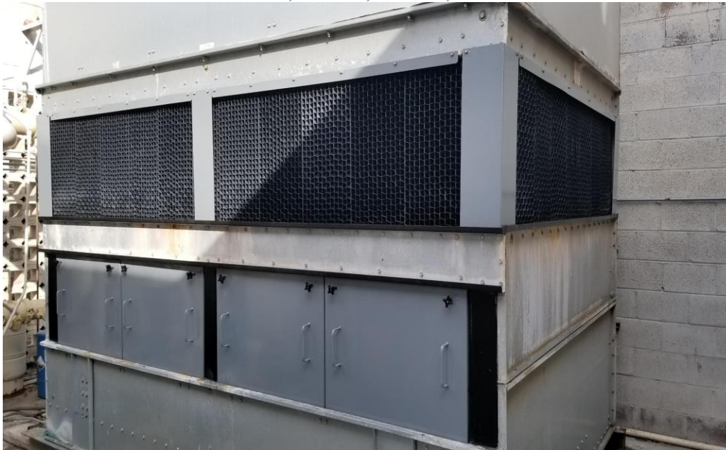
Access Panels, new Knobs, coated trim, and Louvers
