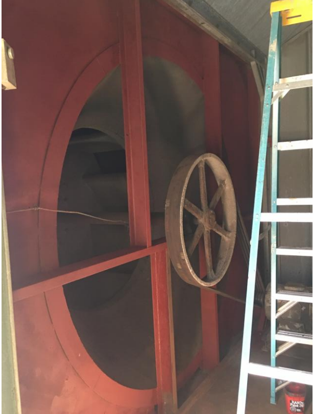
Area around fan housing before, with RCI-A applied then fully coated.
