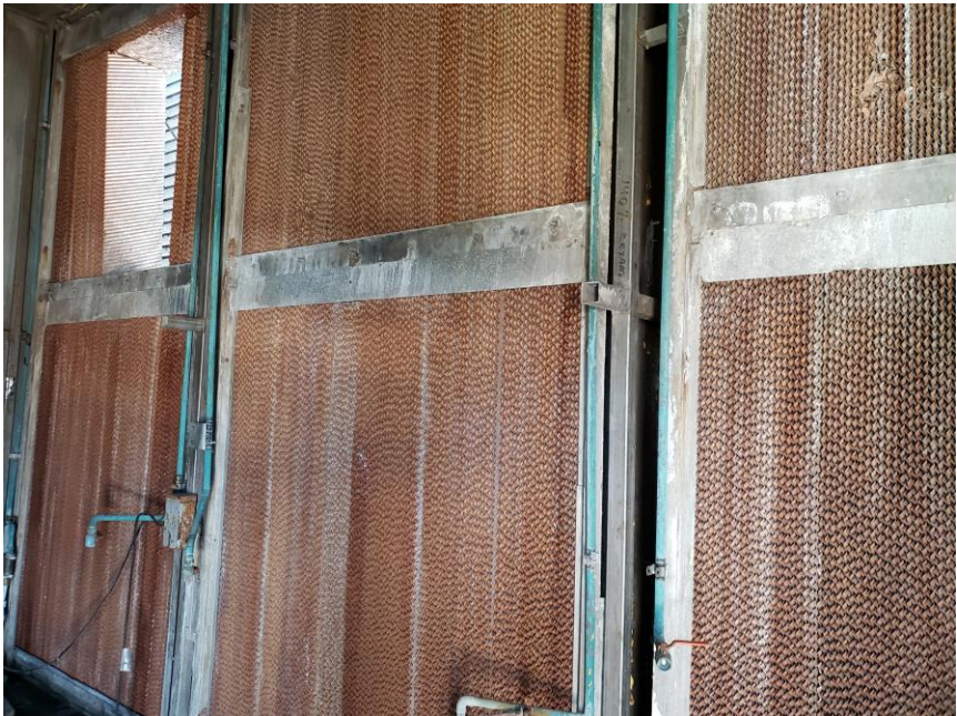
Above is a before and after view of the media area with the drift eliminators installed.
