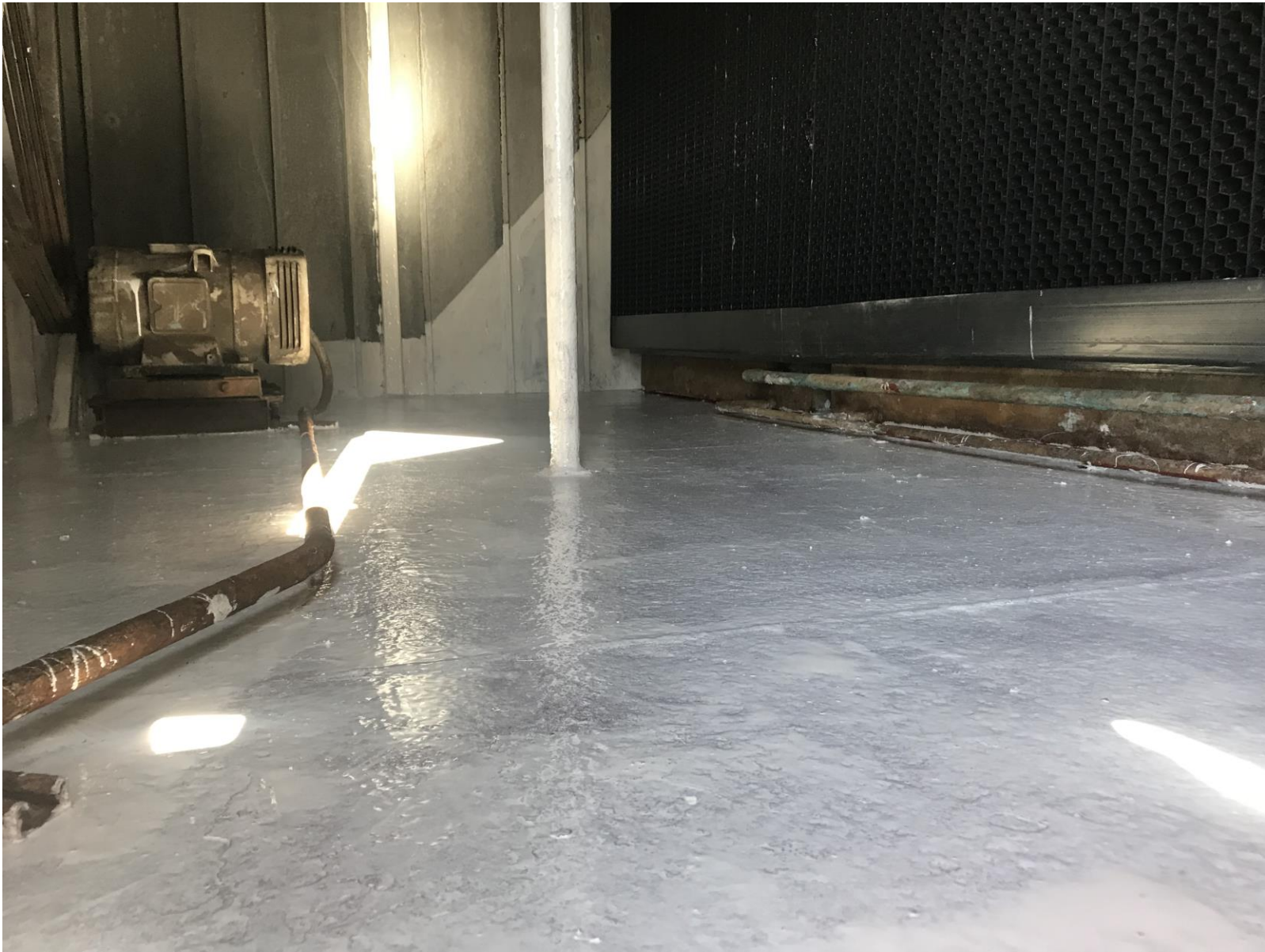
Floor completed and sealed.
