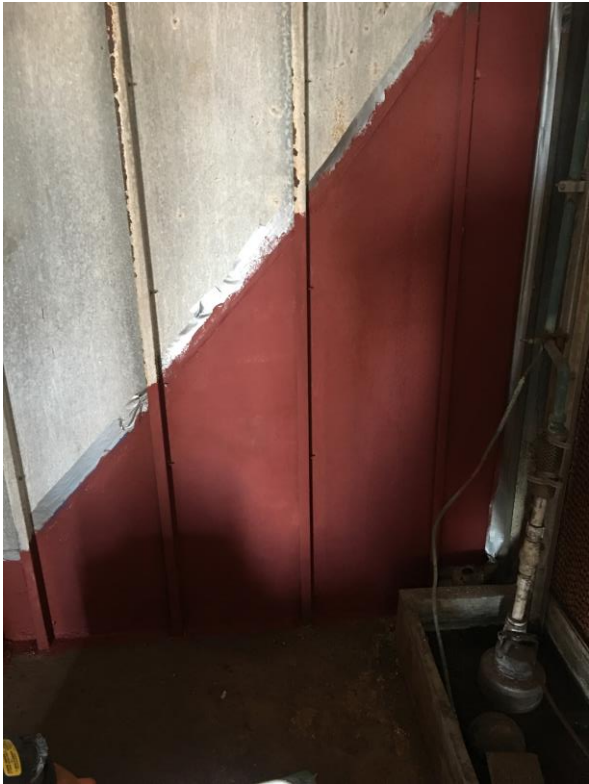
Above is a before and after view of the area around the piping and tight to the wall that we were able to seal.
