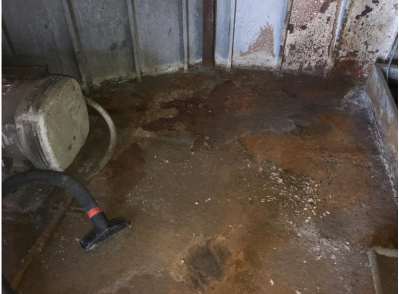
Above are 2 different views of how badly the floor and walls were corroding before.
