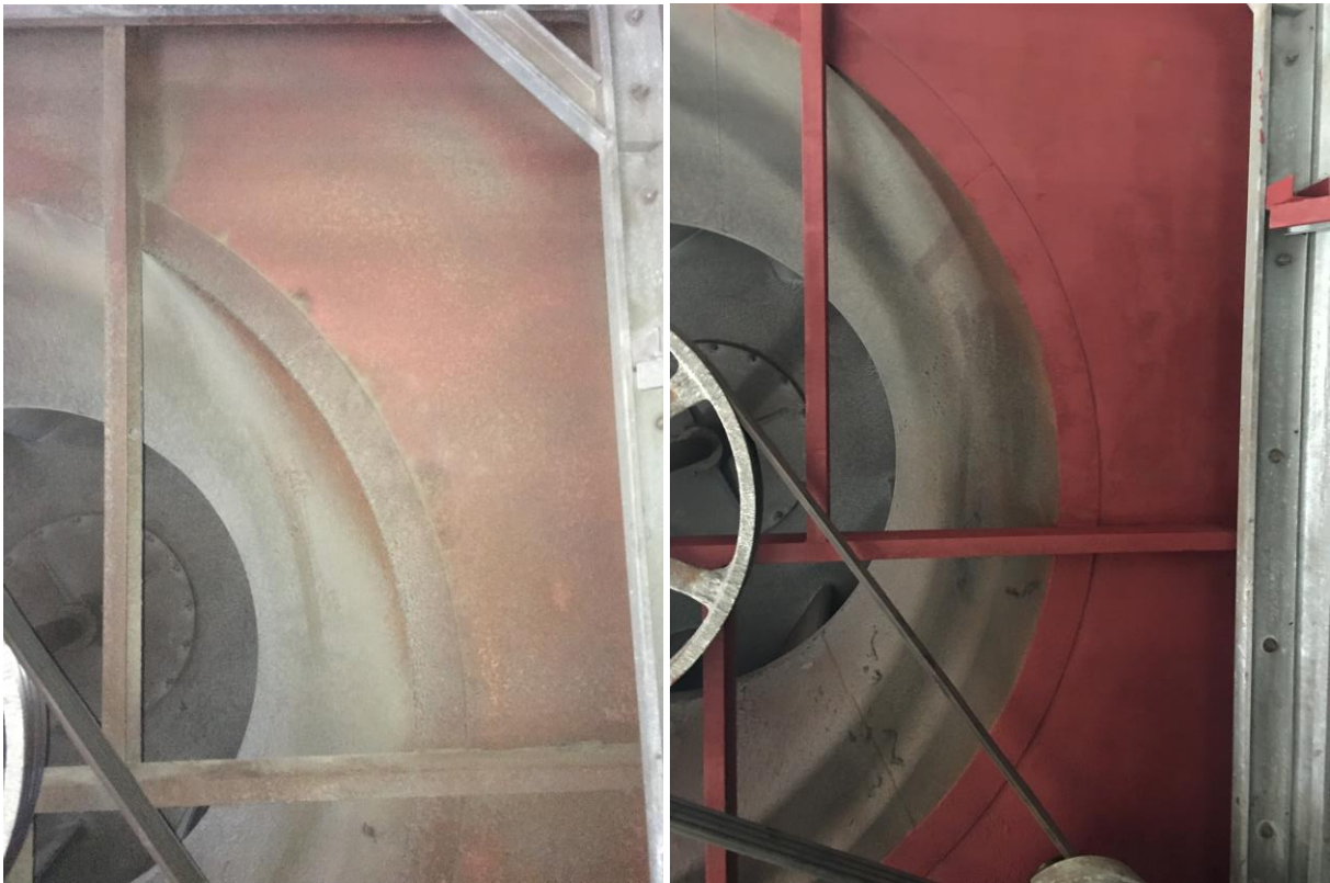
Area around fan housing before, with RCI-A applied then fully coated.
