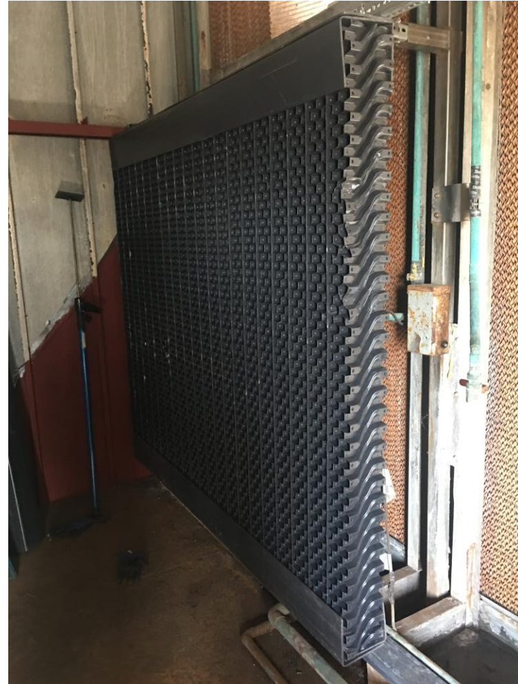
Above are views of the supports built to hold the 6” drift eliminator track in place. Below is a section of the supports installed with drift eliminators.
