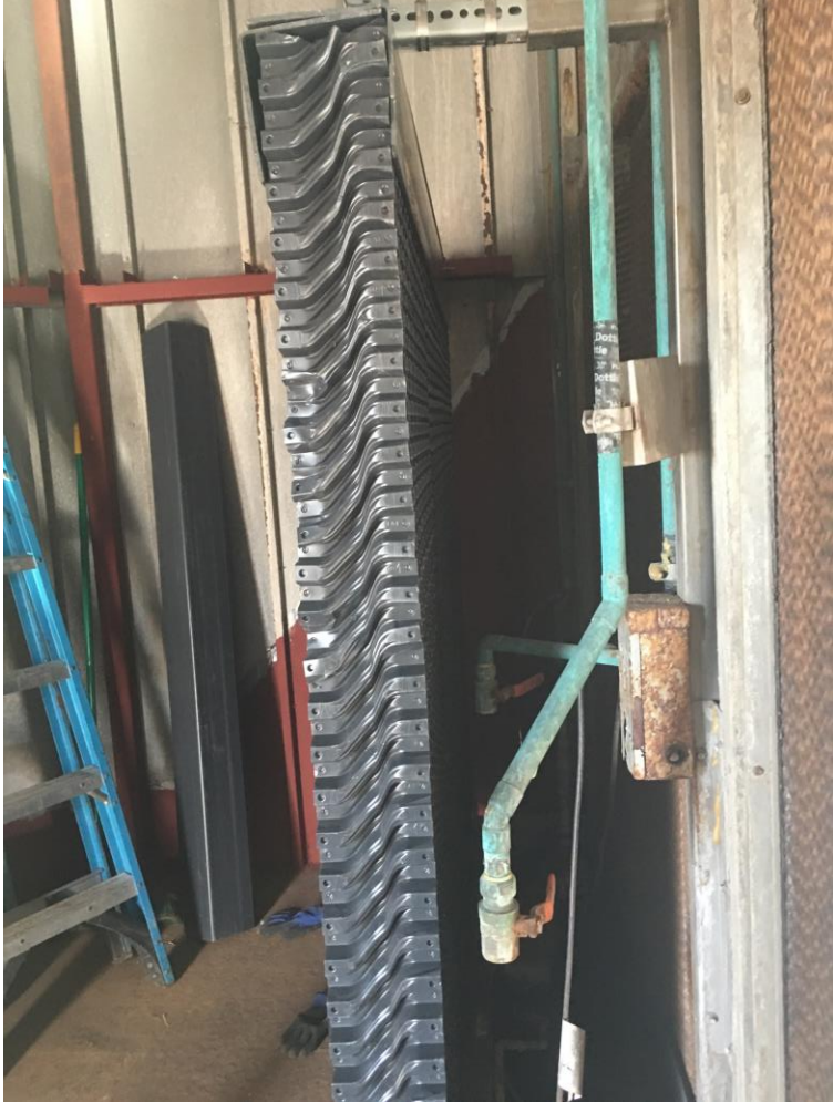
Above are views of the supports built to hold the 6” drift eliminator track in place. Below is a section of the supports installed with drift eliminators.
